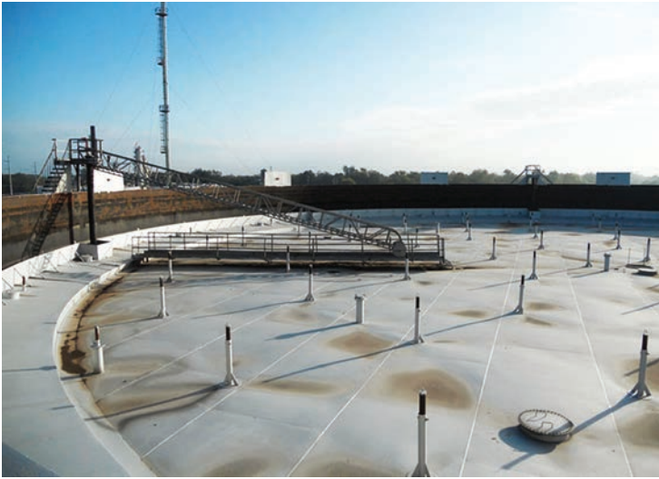
Figure 1. Carbon steel, which is the most prevalent and durable choice for floating roofs, also carries the highest initial capital cost and comes with other potentially significant lifecycle costs. It can also present safe entry issues.
