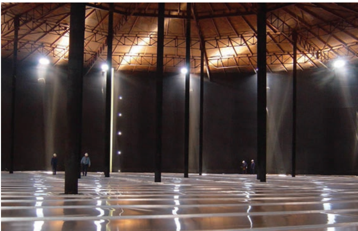
Figure 2. Aluminium internal floating roofs (IFRs) provide a durable, cost effective alternative to traditional carbon steel IFRs.
