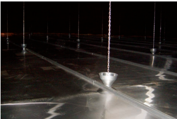
Figure 5. Suspended aluminium floating roofs introduce numerous safety benefits and increase usable capacity over leg-supported roofs.
