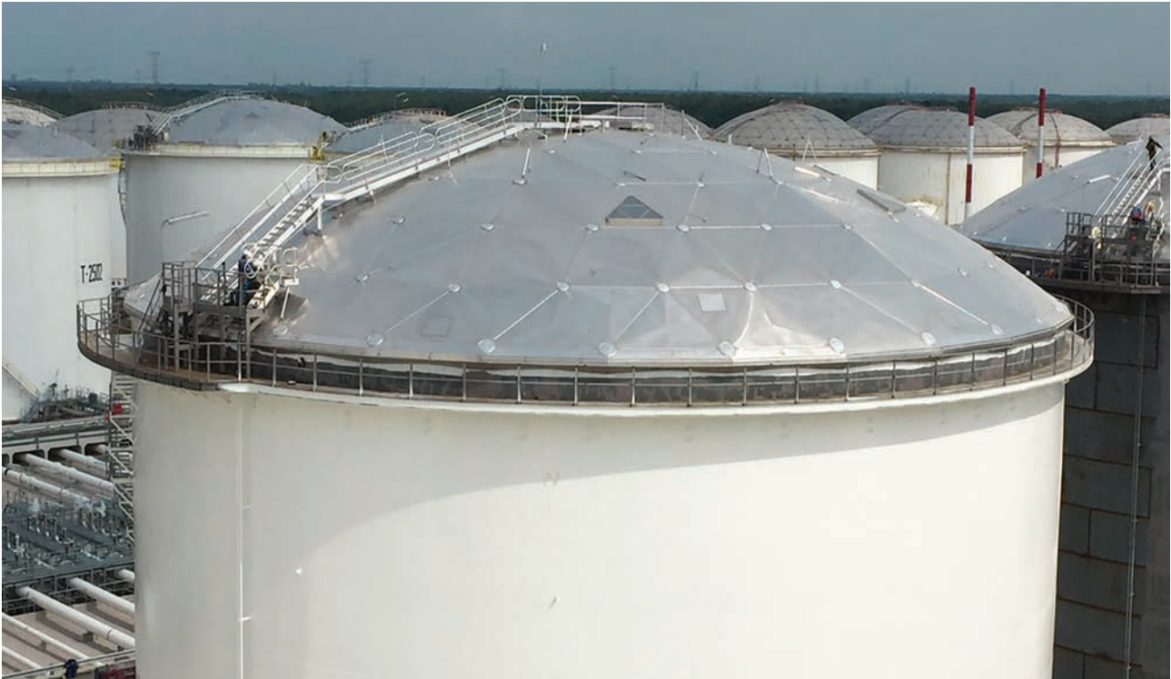
Figure 4. Installation of an aluminium geodesic dome on an open top tank can increase options with respect to IFR selection.
