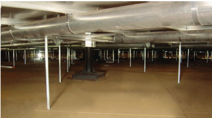
Figure 3. Skin and pontoon designs for floating roofs are the most prevalent in the industry and can be designed to support 1000 point loads.
