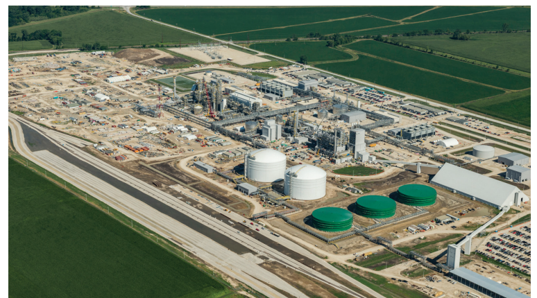
The OCI Iowa Fertilizer facility turned to Matrix for the front-end engineering design (FEED), detail engineering, procurement and construction for ammonia storage and handling systems.
