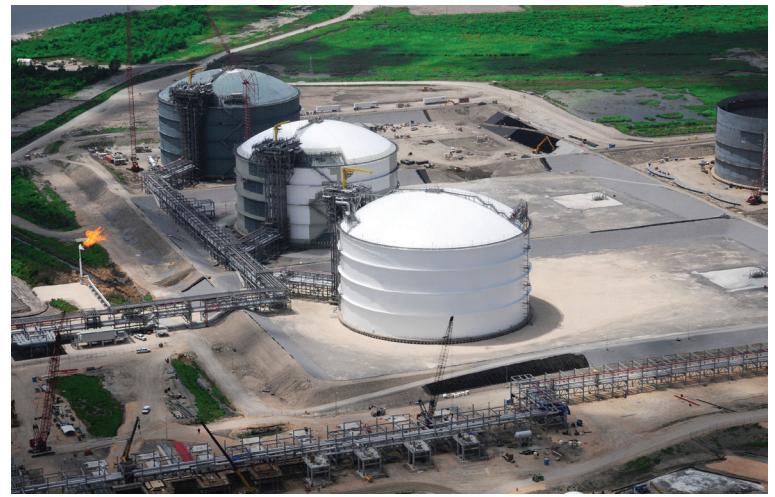
Cheniere’s Sabine Pass, where Matrix provided design, procurement and construction of the LNG storage tanks and their foundations.
