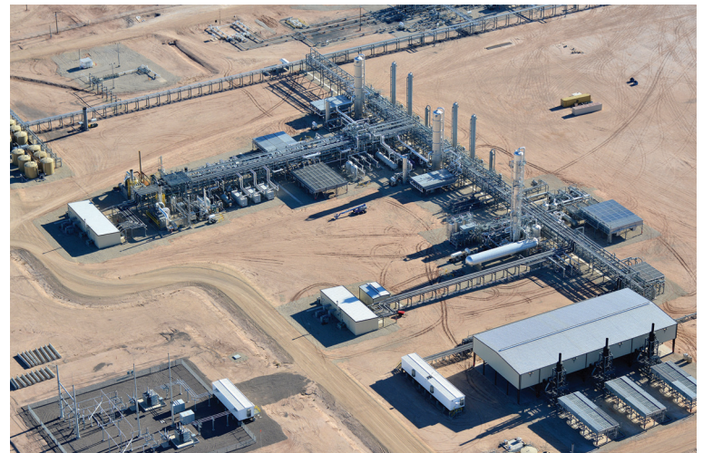
The Red Bluff 200-million-standard-cubic-foot-per-day gas processing facility near Orla, Texas, where Matrix PDM performed the balance of plant engineering, design, procurement and project management.
