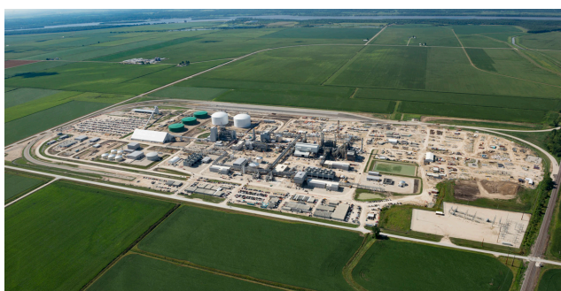
Figure 2. Recently completed state-of-the-art global ammonia production facility in the Midwestern US.
